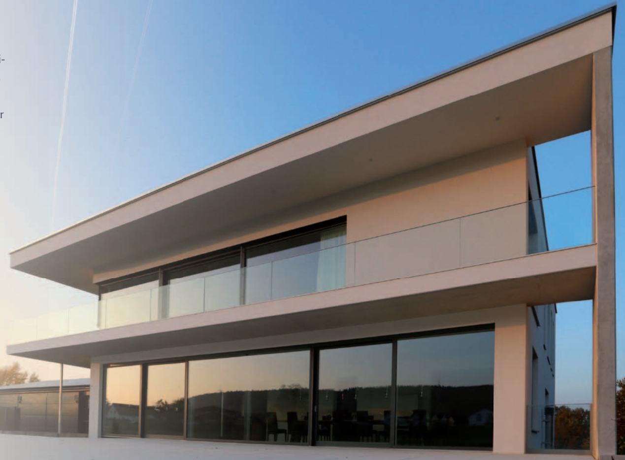
Weingut Rippstein in Sand am Main
